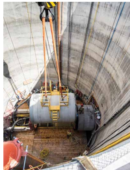
Figure 3. Typical Sunk Caisson Shaft Used in Construction.
