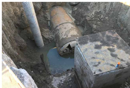
Figure 4. Retrieval of the MTBM in Insitu Shaft Material.
