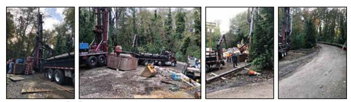
Figure 10. Depressurization well installation
