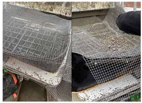
Figure 15. Aggregate captured on screen over grout pump truck hopper
