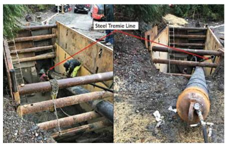
Figure 12. Tremie pipe installed into the borehole annulus adjacent to the product pipe
